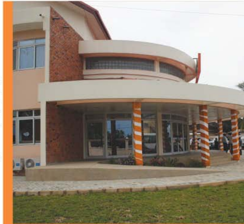
Side View of the Pensioners Recreational Centre
